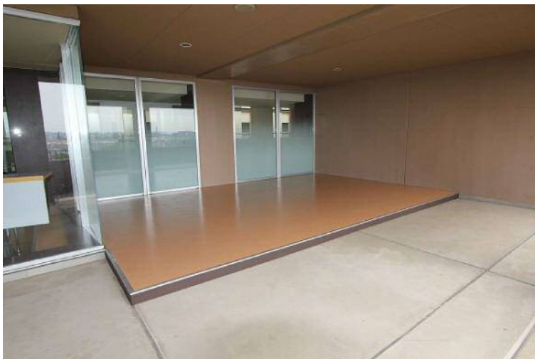
① 研究講義棟5階テラス2改修後 Reserch and Lecture Building 5F Terrace No. 2 After renovation
